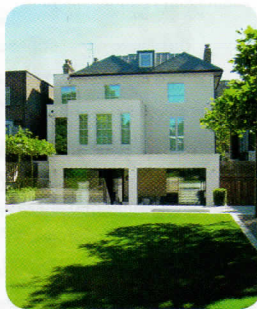
Huge, airy basement No.60 Hole House by James Lambert Architects (020 7608 0833; jameslambertarchitects.com)
